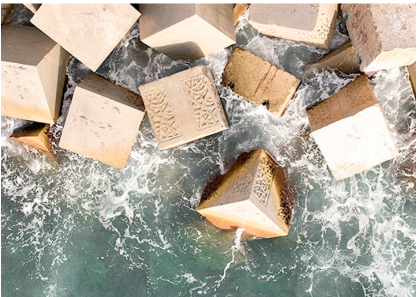
Fig. 91 Port of Cala Rajada Breakwater, ECONcrete. Cala Rajada, Mallorca. ECONcrete
