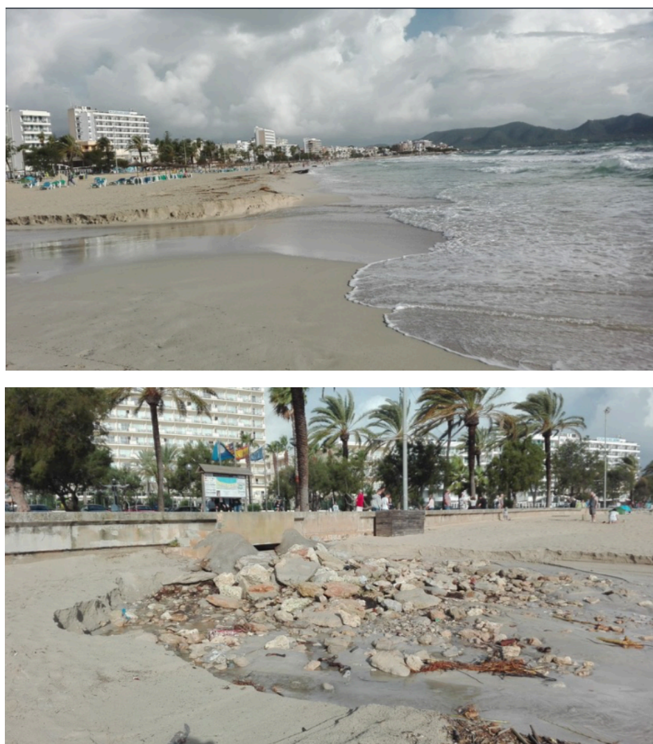
Fig. 5.20. Impact of April 2019 extreme sea storm at CLM. Being one of the most energetic storms from the characterized period, the damage relates with sand transport and accumulation, and accumulation of objects before the promenade.
