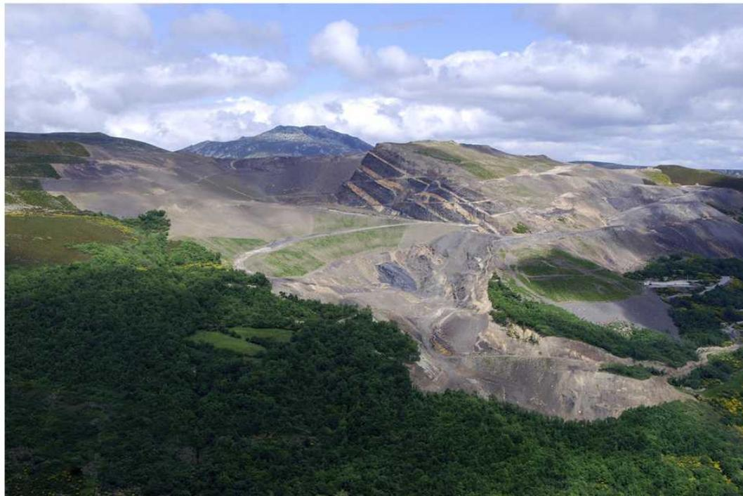
Fig. 3. View of the western end of the surface mine at Feixolín. The restoration did not restore the original topography, leaving a large pit on the hillside and an escarpment exposing porphyry outcrops between the layers of coal. The mining is in a valley that is home to endangered species such as the brown bear and Cantabrian capercaillie.
