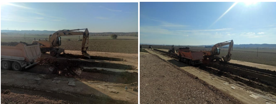
Figura 7. Zanja balsa de upgrading
