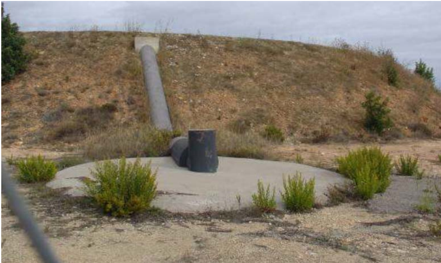
MAR borehole associated to an Irrigation pond
