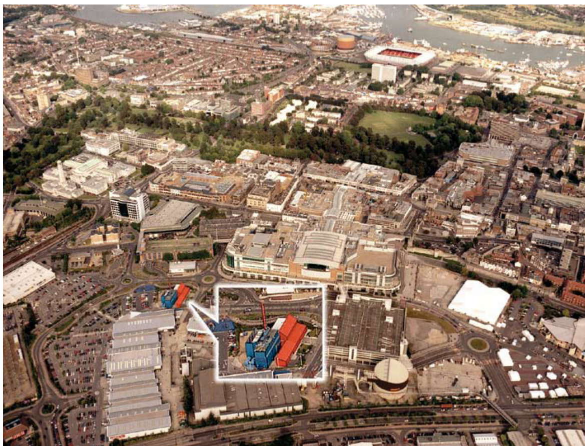
Figura 5: Southampton (Photo: SCC/Utilicom) (Fuente: Southampton Geothermal Heating Company Ltd.)
