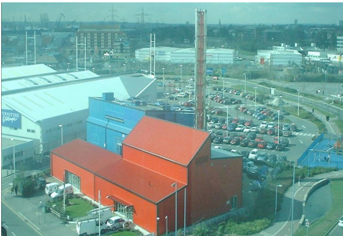
Figura 4: La central energética de Southampton: The Red and Blue heat station. (Photo: SCC/Utilicom) (Fuente: Southampton Geothermal Heating Company Ltd.)
